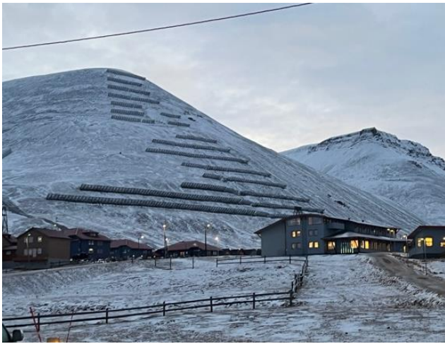
Structural protection measures at Sukkertoppen (Photo: E. Albrechtsen)
