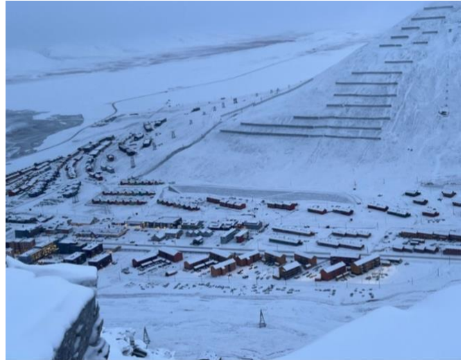
Longyearbyen with structural snow avalanche protection measures (Photo: E.Albrechtsen)
