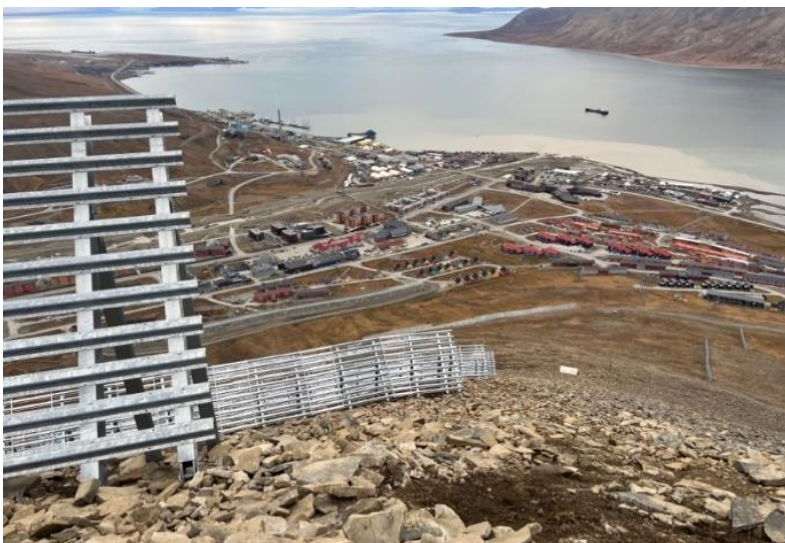
Supporting structures, catching dam and snow fences seen from the upper part of Sukkertoppen. Photo: Eirik Albrechtsen
