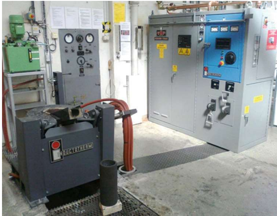
Fig. 4 Induction furnace used for smelting-reduction experiments
